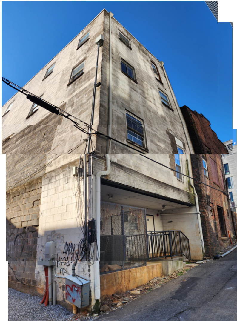
3 SE VIEW FROM SERVICE ALLEY
